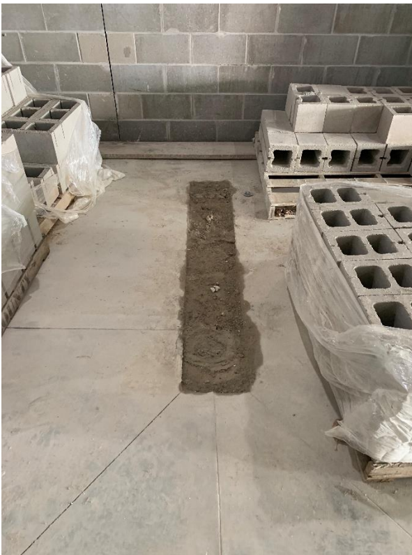
29. Area 3 – Recessed slot drain rough opening at receiving.
