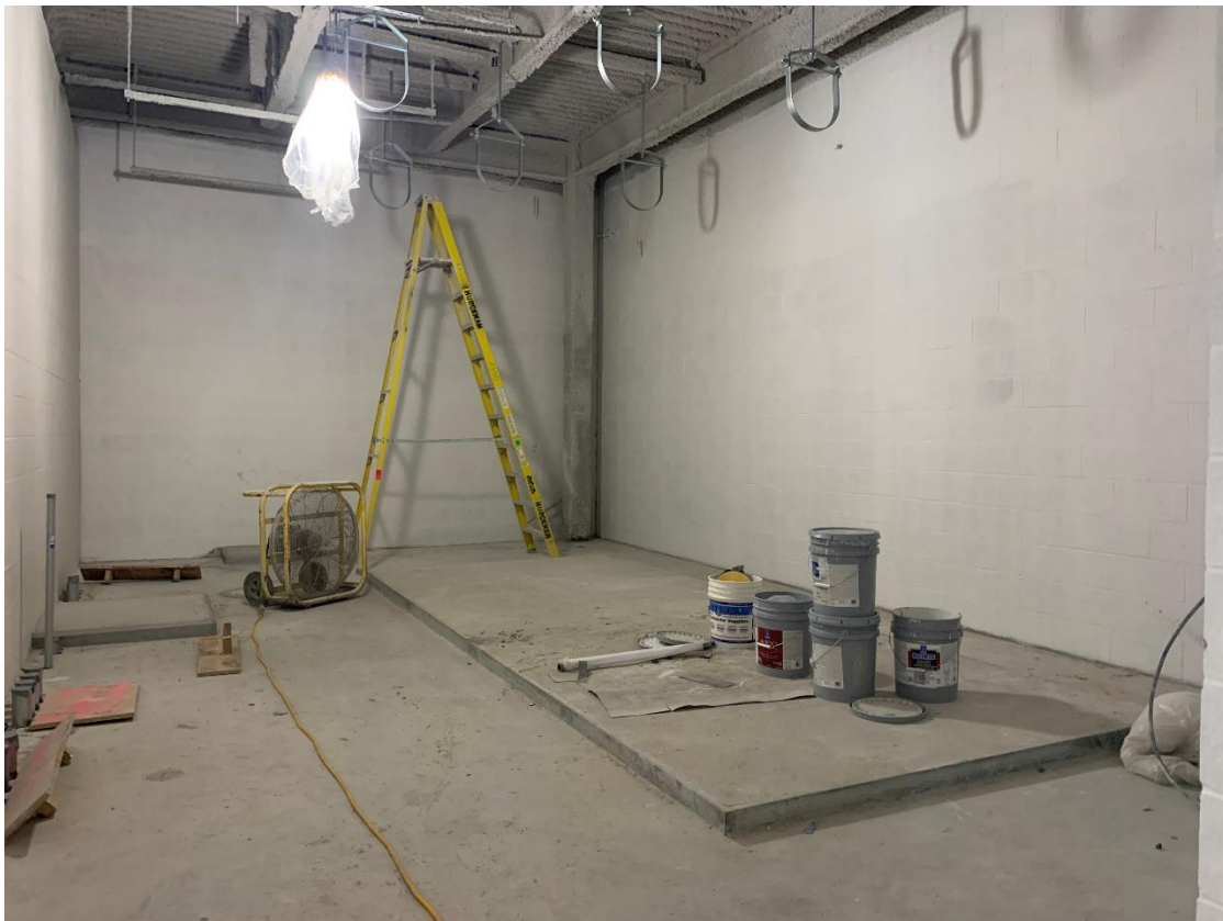
12. Area 6 – Second floor pump room wall primer in progress.
