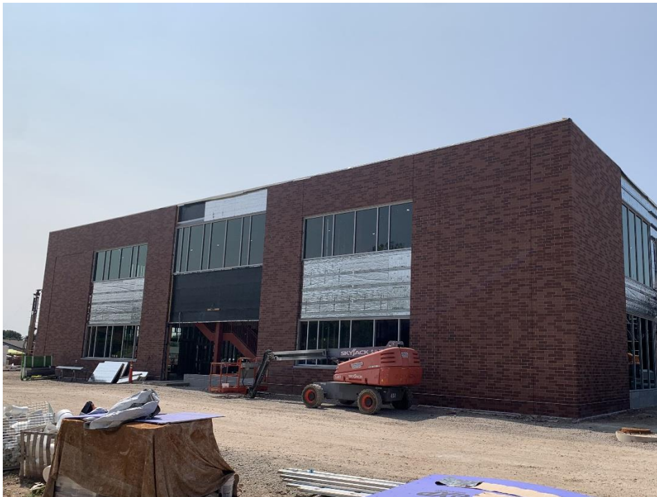
20. Area 5 – Exterior brick and cast stone installed. Exterior board insulation and girt system installation in progress.
