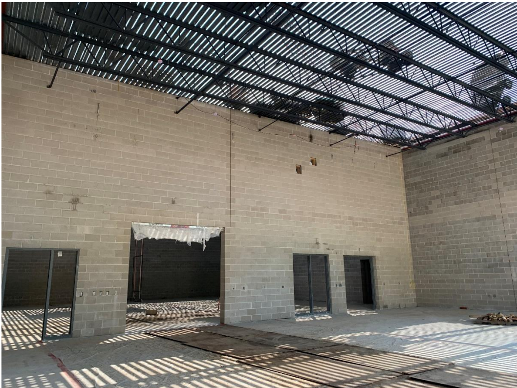
31. Area 3 – Acoustic decking in tech ed. Roof insulation, hollow metal frames, and plumbing installation in progress.
