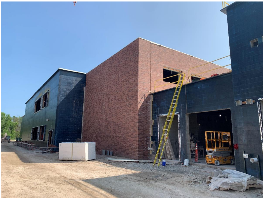
33. Area 3/4 – Exterior brick, AVB, and Window weather proofing membrane installation in progress.
