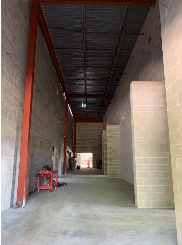
31. Area 3 – Acoustic decking in tech ed. Roof insulation, hollow metal frames, and plumbing installation in progress.
