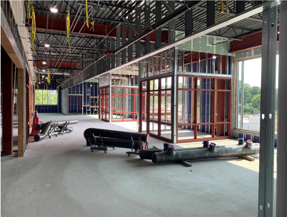
10. Area 5 –In wall plumbing, blocking, and insulation installation in progress.
