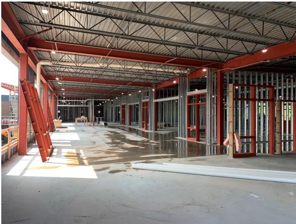
25. Area 4 – Interior metal stud and hollow metal framing installation in progress.
