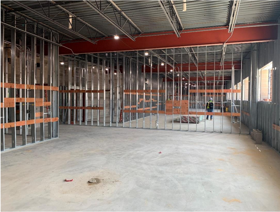
25. Area 4 – Interior metal stud and hollow metal framing installation in progress.
